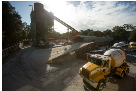
Concrete plant in Alexandria
